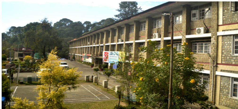
Main Block of the Zonal Hospital at Dharamshala.
